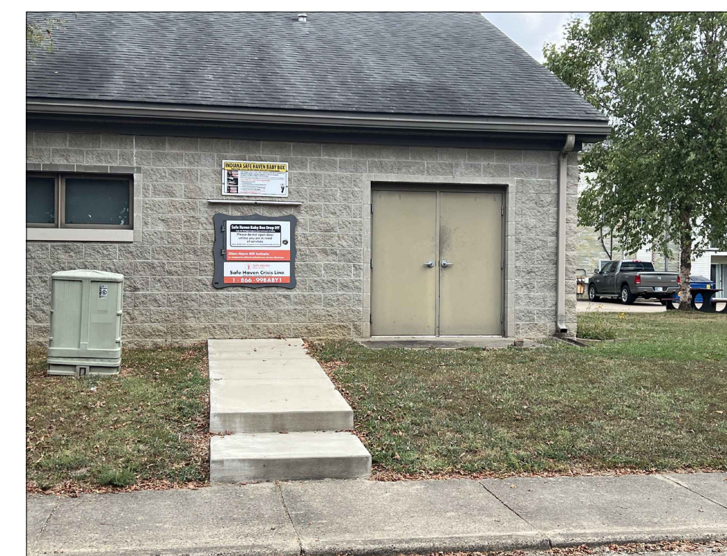
Existing Baby Box exterior installation for reference.
