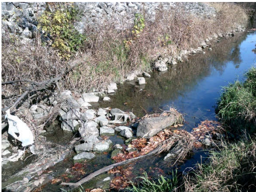
Examples of rip rap blockages and debris at various points along the channel
