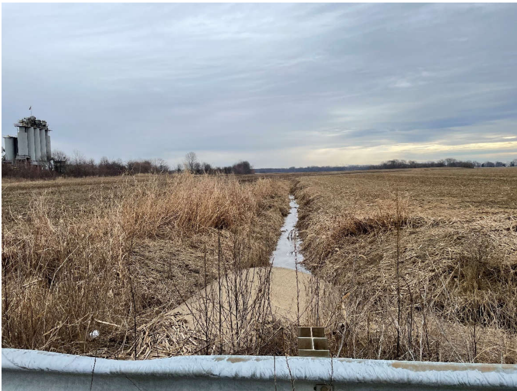
Eagle Slough east of Green River Road
