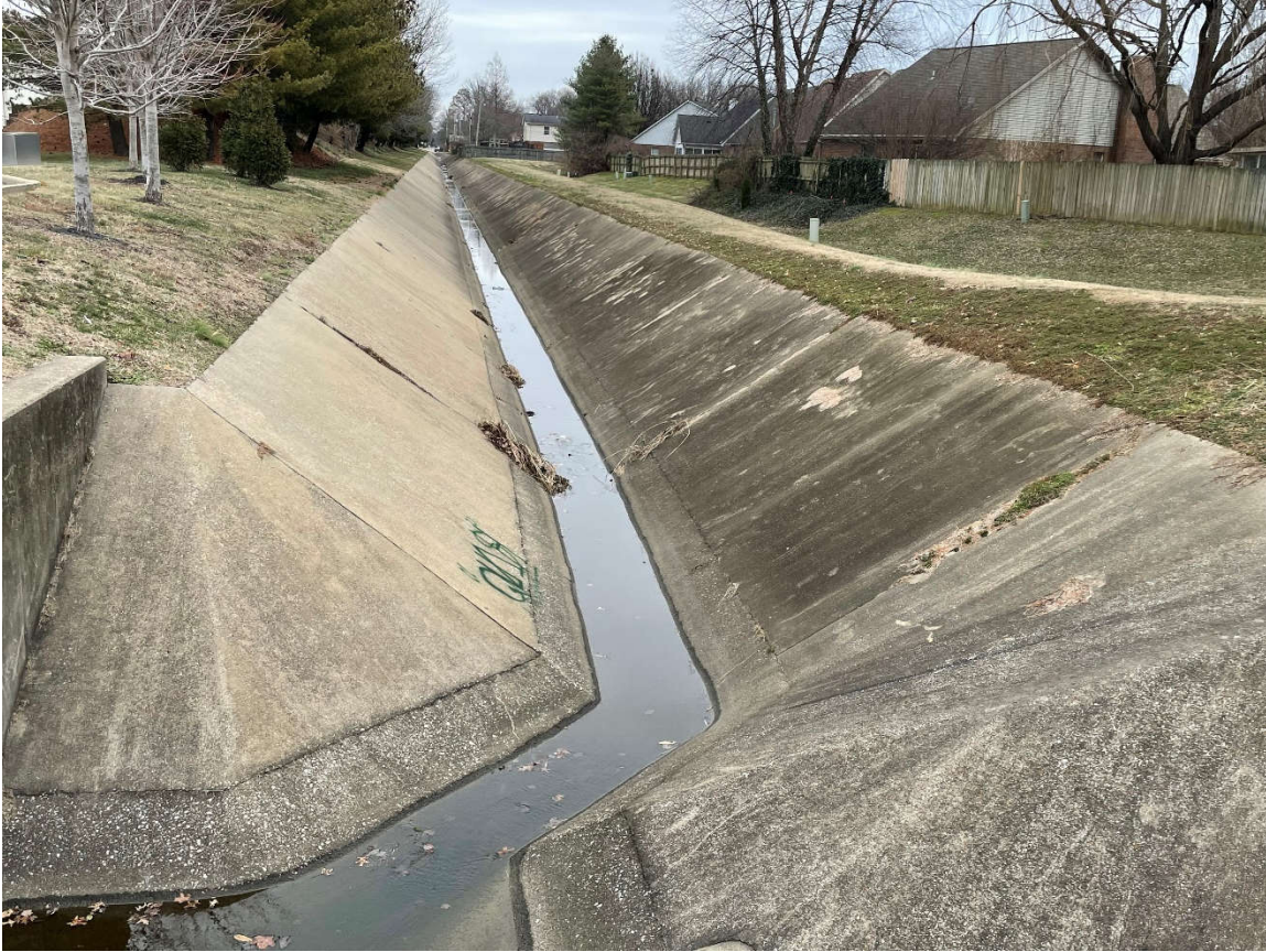
Bonnie View Concrete Ribbon Liner
