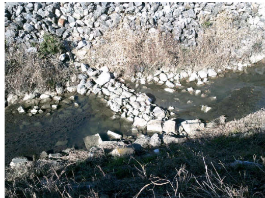
Examples of rip rap blockages and debris at various points along the channel
