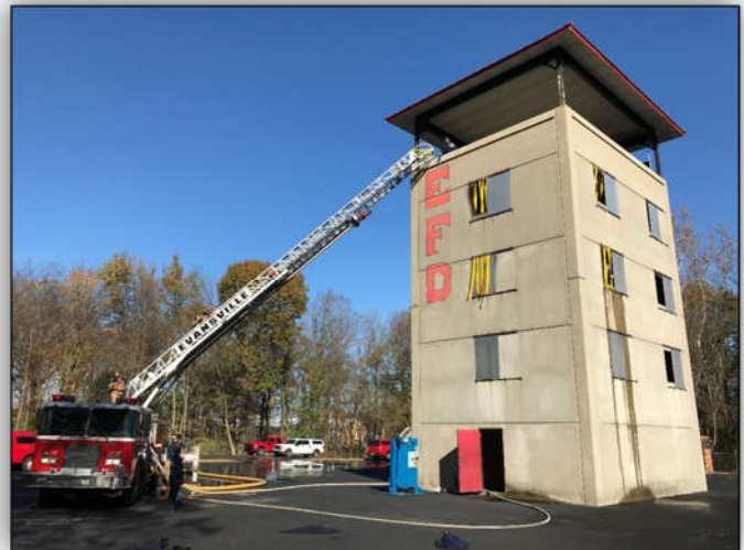
Five-Story Training Tower Building
