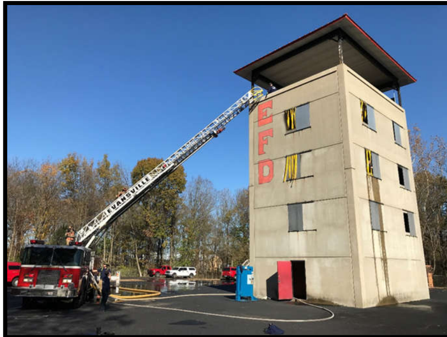
Above: Five-Story Training Tower Building.
