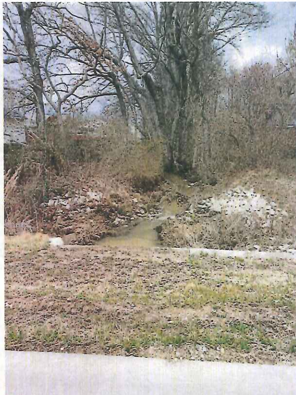
March 7, 2022 – looking north at ditch running between Fenway Park subdivision and Valley Estates subdivision
