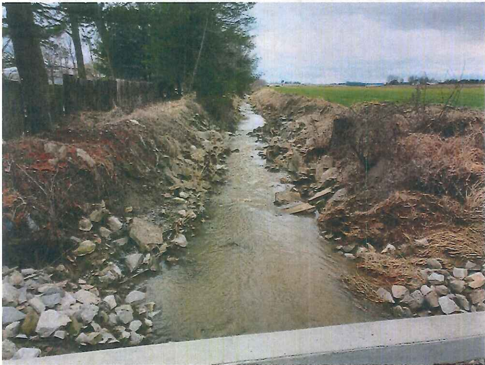
March 7, 2022 - ditch downstream of Korff Road looking west
