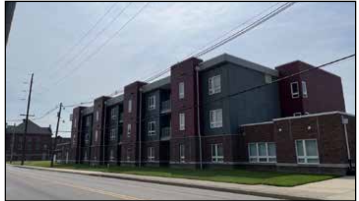
A larger apartment complex along Garfield Street
